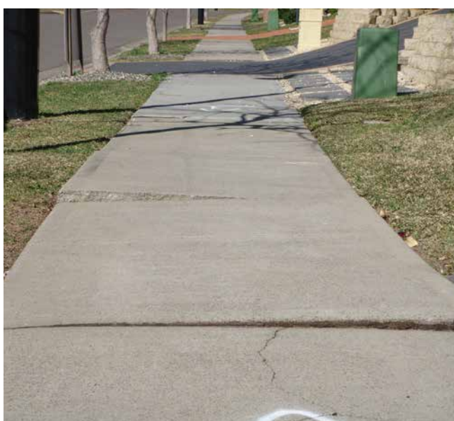
Fig 2.1.4 - Pavement damage caused by shallow rooting.
