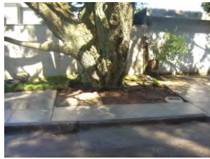
After: Sidewalk opened up around tree
