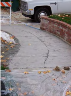
Poured in place rubber Sidewalk
